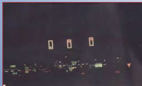
Figure A-4. Retro-reflective Backplates (Nighttime)
