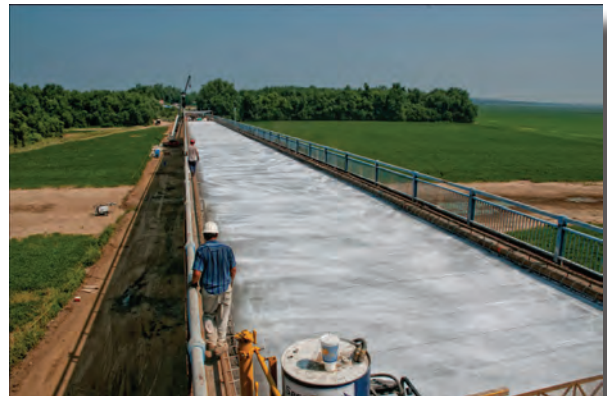
New completed bridge deck
