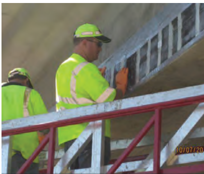
Application of CFRP Rod Panels
