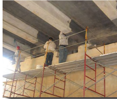
Application of SFRP fabric
