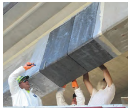
Application of CFRP fabric
