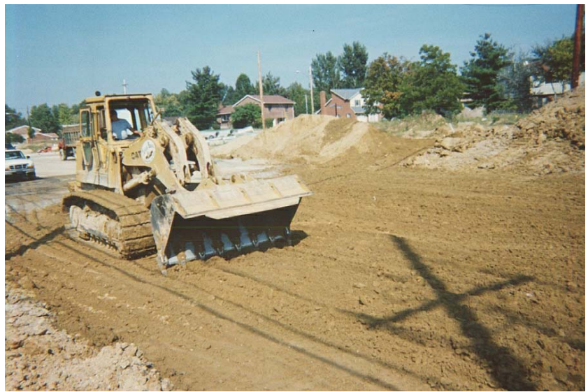
Figure 10. Mixing stockpile hydrated lime-soil with a front end-loader, Stevenson Road.
