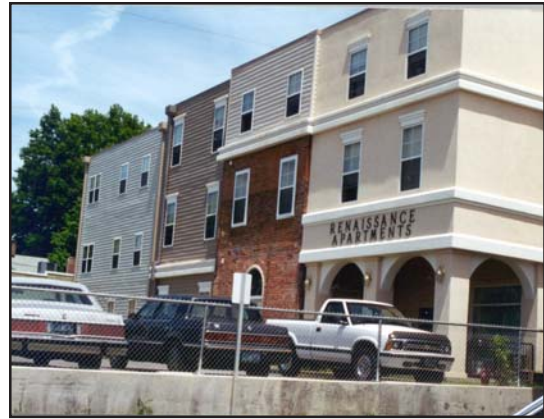
Renaissance Apartments in downtown Irvine with retail spaces below.
