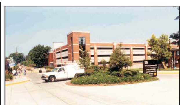
Part of Hilltop Avenue on UK's campus in Lexington was closed off to thru-traffic and a single-lane roundabout installed. It allows traffic to safely enter and exit the permit-only parking structure and also allows those drivers who don't realize it is a permit-controlled structure until they're there to easily turn around and not have to back out.
