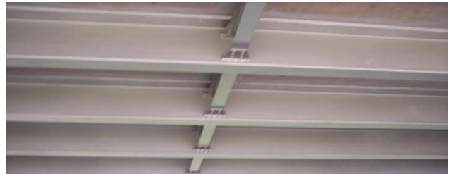
FIGURE 6: College Park Dr Bridge 2008, LADOTD
