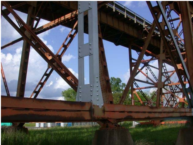
FIGURE 3: US 190 Bridge 2003, LADOTD
