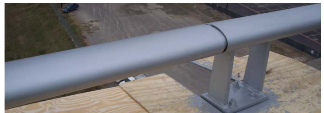
FIGURE 10: Railings After Rust Grip® 2008, TXDOT
