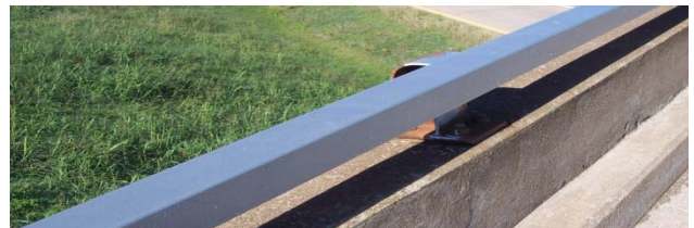
FIGURE 8: Railings After Rust Grip® 2008, OKDOT
