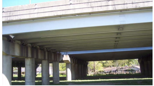
FIGURE 5: College Park Dr Bridge 2008, LADOTD
