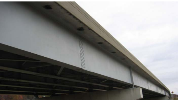
FIGURE 13: US Highway 52 Vicksburg, MSDOT
